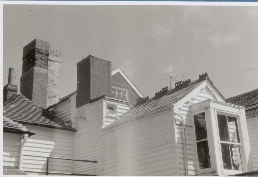
REAR VIEW, seaward side. Evidence of poor maintenance, superficial repairs. Roof leaking, gutters and pipes rusted. Projecting bay decaying, weatherboards replaced with mineralised felt. Unsightly water tank and obsolete chimney stack. This room could provide excellent galley and storage space
