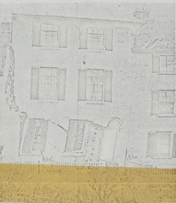
Spring House, with gaping crack in outer wall and displacement of ground floor rooms.
