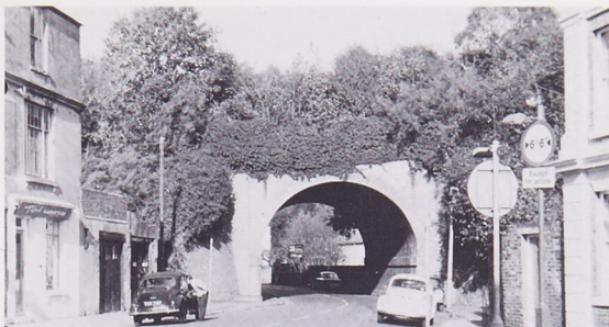
The old railway bridge in Horn Street
