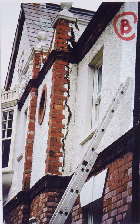
Above: Cracks re-open. 'Stopped' June 2005
