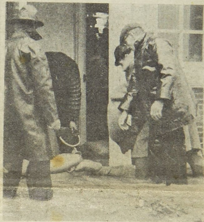
Sandbags are laid at the doorstep of a Sandgate house in an effort to keep out the floodwater which swept through the streets on Saturday.
