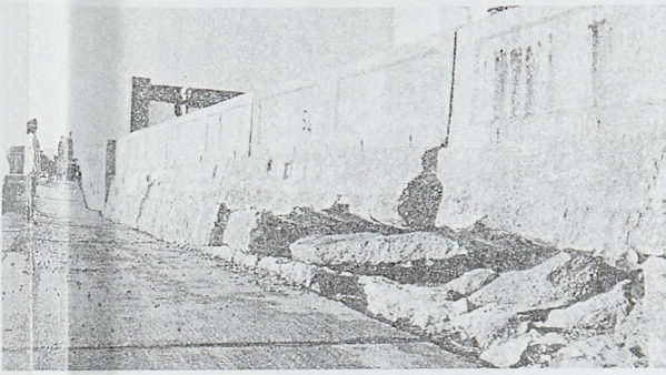
● Concrete crushed like paper
