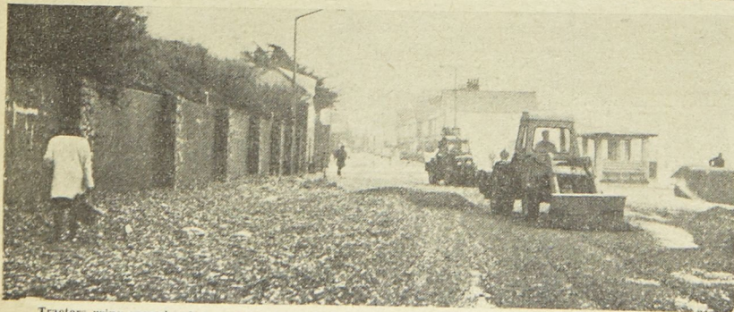
Tractors using snowplough equipment start the long task of shovelling away hundreds of tons of shingle.
