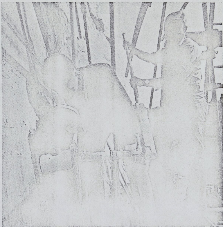
Fig. 7. Prestressing rock bolt fitted with optical load cell for underpinning of chalk cliff at Dover, Kent
