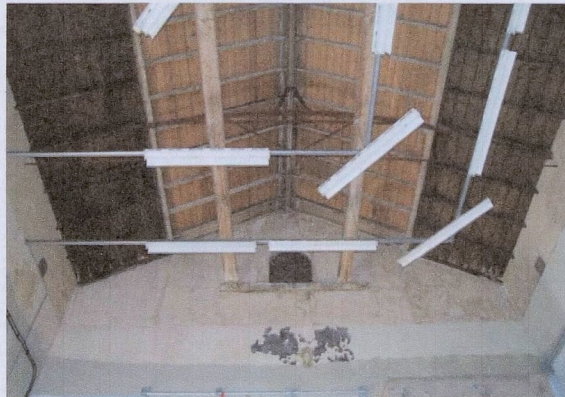
Figure 18: Interior view of the Racquet Court with lattice steel girders likely installed by the Royal Engineers as an experimental roof structure.
