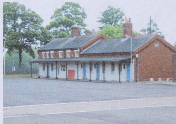
Figure 30: View of the Guardhouse at the northern entrance into Napier Barracks.
