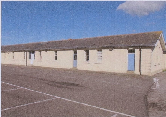
Figure 15: View of Grade II listed Concrete Barrack Block I; south elevation.
