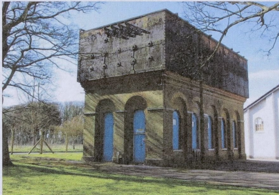
Figure 20: Water Tower south of the Grade II listed Racquet Court.
