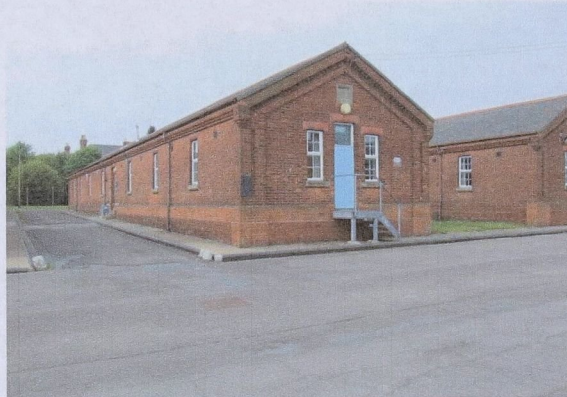
Figure 29: Row of barrack blocks in Napier Barracks. The north easternmost barrack block closest to the north entrance forms a police house.
