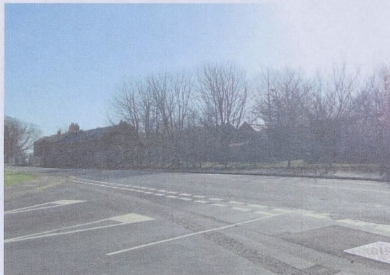
Figure 28: View of Somerset Barracks from North Road where the Officer's Quarters, Mess and Quartermaster's Quarters lie.
