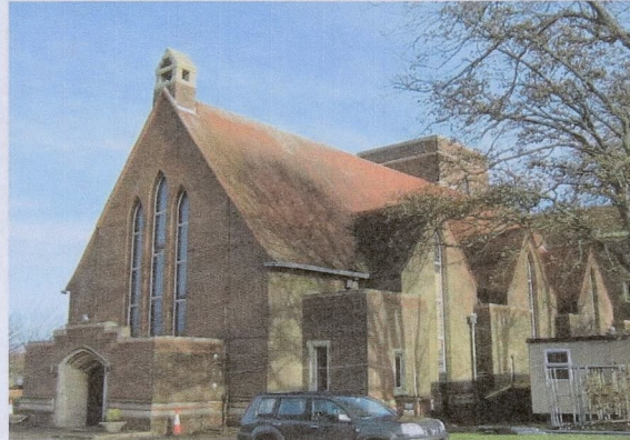
Figure 13: The Grade II Listed Garrison Church of St Mark's was symbolically built during the Second World War.
