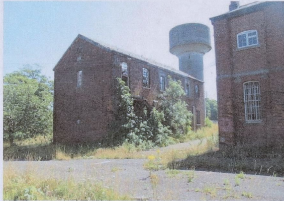
Figure 23: View of the derelict state of buildings within Risborough Barracks.
