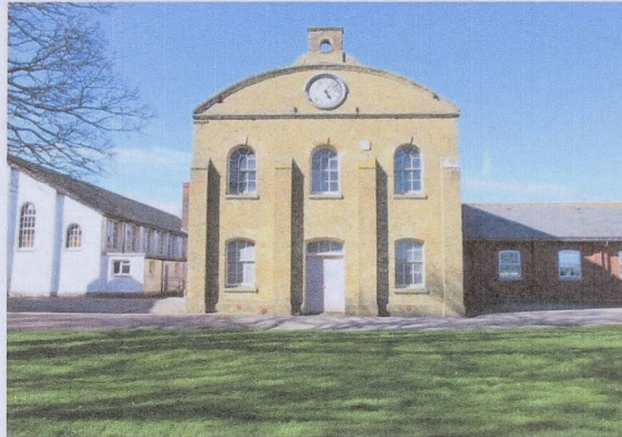
Figure 17: View of the Racquet Court's east end gable featuring an round-arched brick parapet with original clock and bell-cote. Such architectural details enhance its architectural interest.
