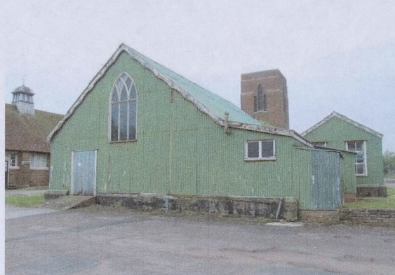
Figure 27: Disused Church/Hall which appears to be in an advanced state of decay.
