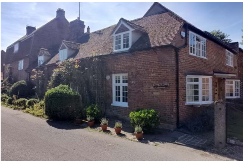
Ivy Cottage and Forge Cottage
